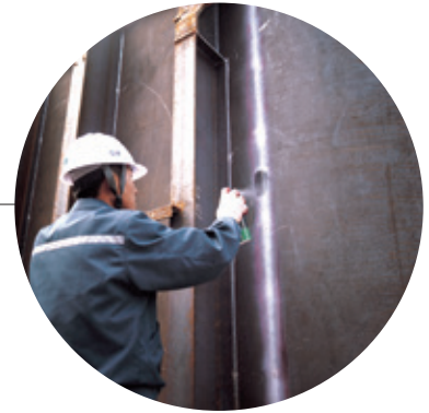
Non-Destructive Test on Transformer Tank
