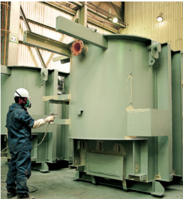
Painting of Tank
